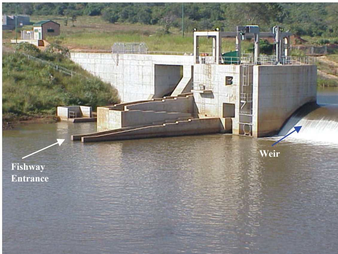
Plate 8.1: A view of the three sections of the Xikundu fishway
