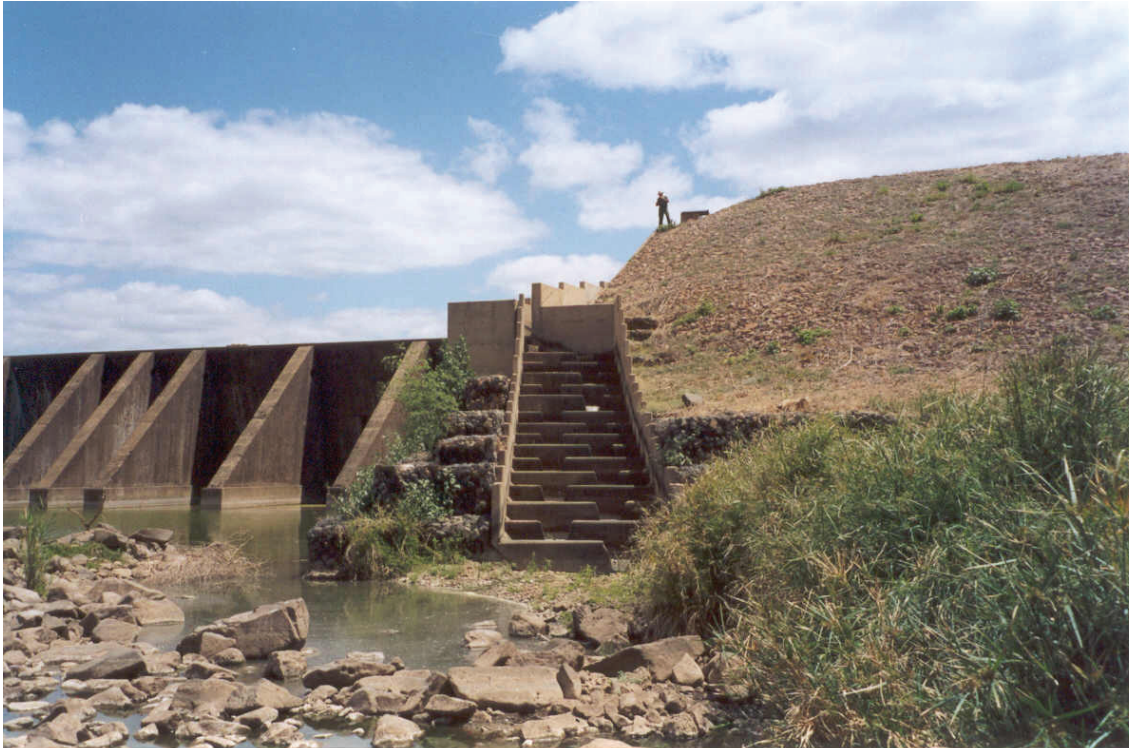
Plate 3.1: View looking upstream at the Kanniedood fishway on the Shingwedzi River in the KNP during low flow conditions.
