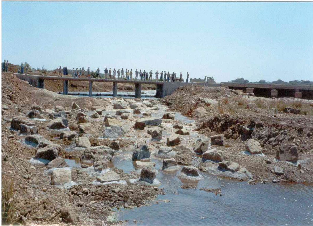
Plate 3.6: Lower Sabie bridge Rock-ramp fishway at commissioning in October 2001.
