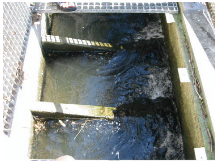
Plate 7.4: Grating removed to show pools and baffles inside Nhlabane Fishway.
