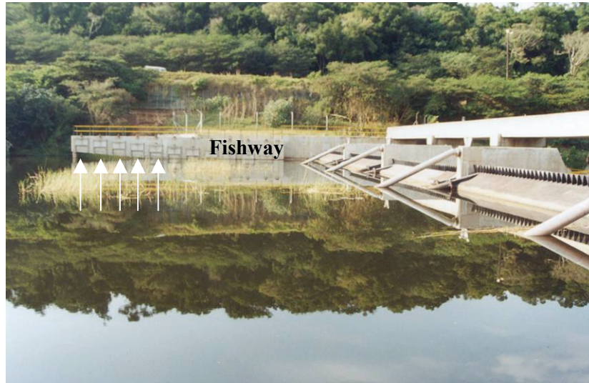
Plate 7.3: Upstream view of Nhlabane weir and fishway exit during low lake level. Arrows indicate positions of exposed exit ports/inlet sluices.
