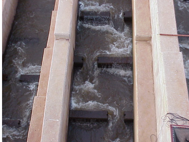
Plate 8.3: Flow pattern in the fishway
