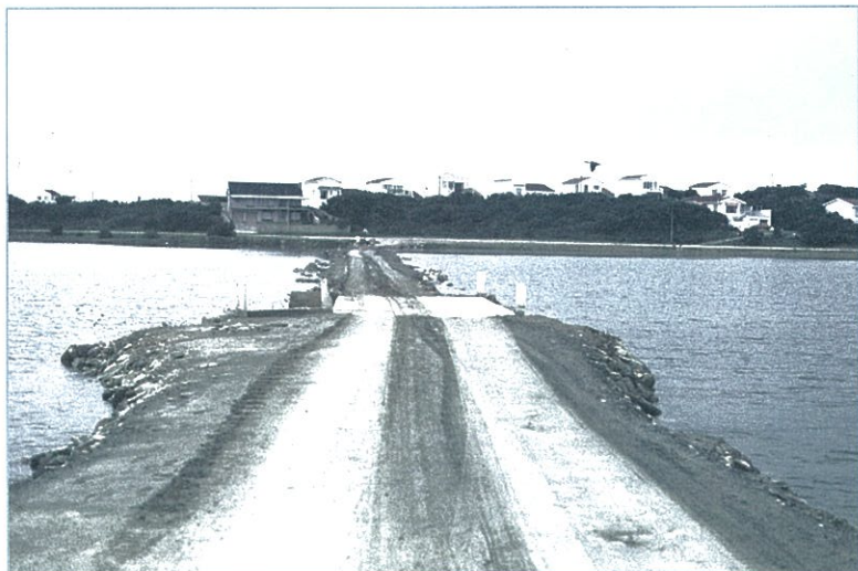
Causeways like this one at the Seekoei can completely alter sedimentary processes in estuaries (DEAT)
