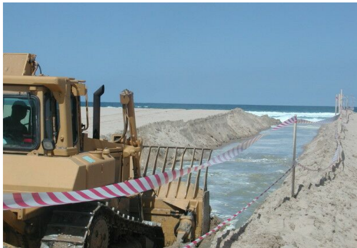
Opening an estuary mouth artificially can rapidly and radically change the system (Piet Huizinga)
