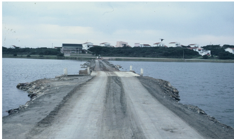
Construction of this causeway fundamentally restricted the water flow in the estuary (DEAT)
