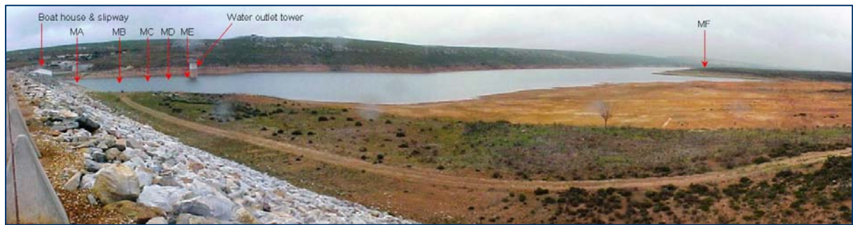
Figure C-2b The Impofu Dam, showing sampling points for this study (ME – at outlet, MF – 1 km upstream of outlet)
