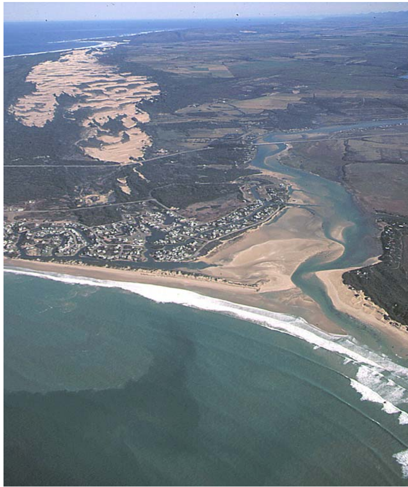
Figure G-2 Aerial view of the lower reaches of the Kromme Estuary. The building of two large reservoirs in the catchment has led to less frequent floods that are capable of removing sediment from the estuary. Sand is mostly of marine origin through the mouth, although some is deposited in the estuary via the Sand River flowing at times from the extensive dunefield seen on the left of the picture. This dunefield used to deposit sand where the marina is currently situated. Erosion along the dune complex separating the marina from the sea is also clearly visible.
