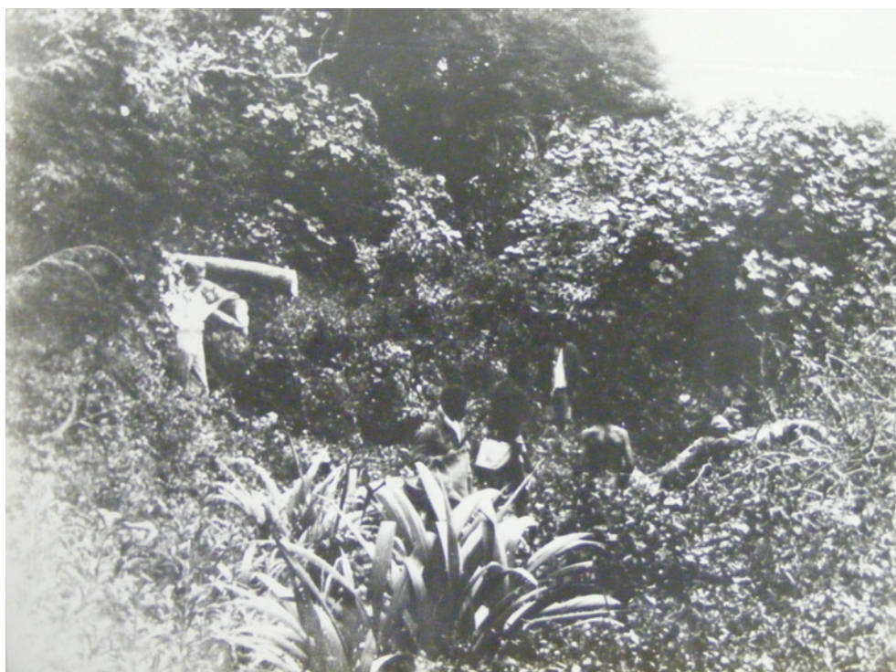
Photo 15. Cutting a path through Mapelana forest, 1929. See photo No 11. (Photo: Woods, 57).
