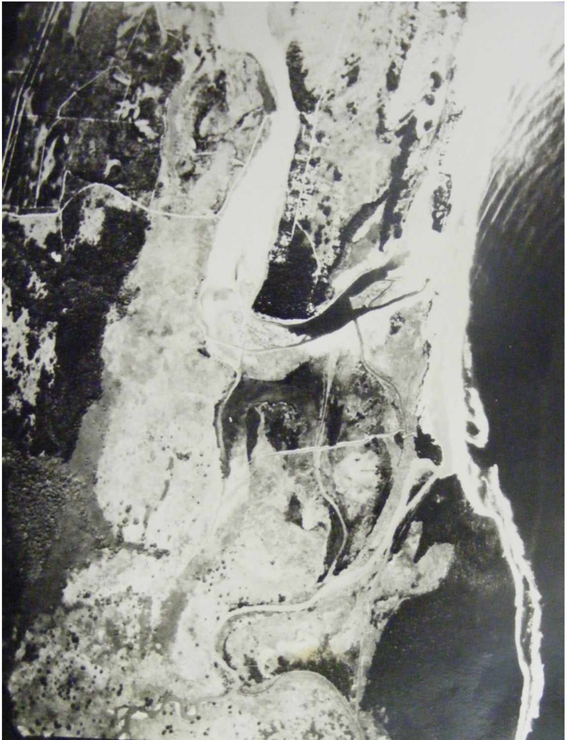
Photo 10. Trigsurvey Photo No. 2271 of Job 442 of 1960. Considerable dredging had taken place, the Levee completed and a two span bridge erected.
