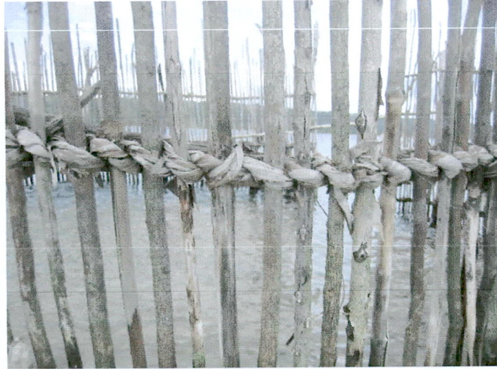
Figure 3. Kosi Bay fishtrap ljeli terminal basket wall showing traditional Ugude ( Strelitzia nicolae ) binding, note large gaps between sticks.
