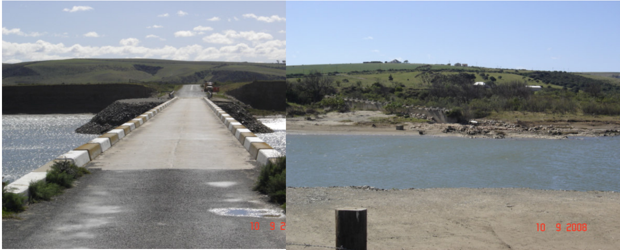
Plate 7.3 The existing low bridge over the Gouritz estuary with stabilizing materials that alter the flow dynamics (left) and the remnants of the original bridge washed away by the 1981 flood waters (right).
