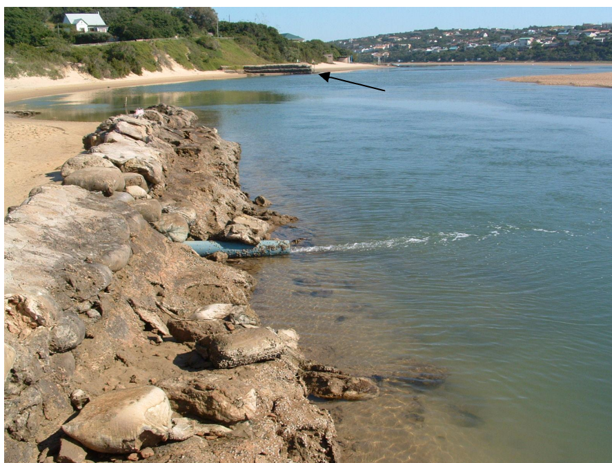
Figure 3. Upstream view of the western bank of the Bushmans Estuary, showing the position of the discharge pipe at the Deacon sandbag wall. In the background, further upstream is the gabion wall (arrow), which is the proposed location of the seawater inlet pipe.
