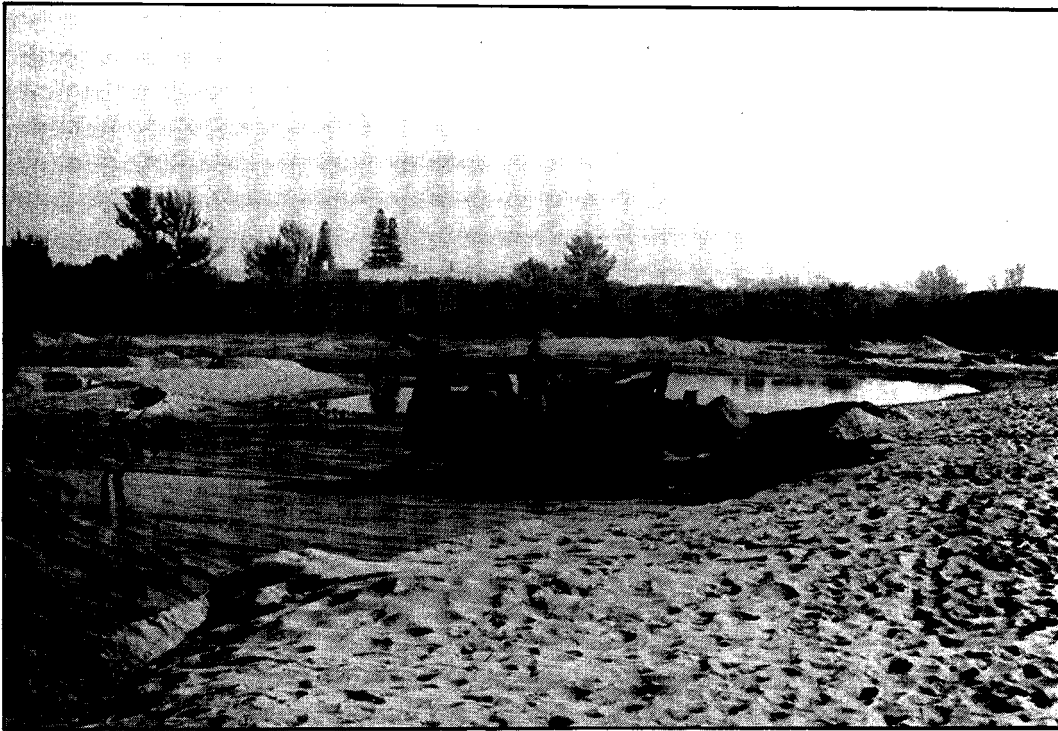
(Plate 2): Restoration of the Sipingo Lagoon partially depends on increasing the tidal prism by excavating sand from the mouth region.
