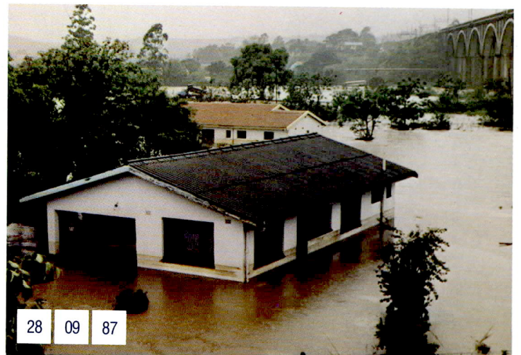
NB: PEAK FLOOD LEVEL MARK ON THE HOUSE
