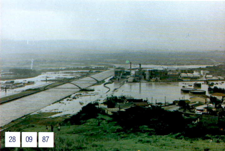
MLAZI CANAL AND INUNDATED AREAS: NEAR PEAK DISCHARGE
