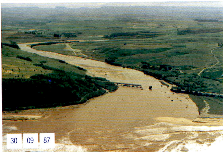
DAMAGE TO THE ROAD BRIDGE NEAR MOUTH OF MDLOTI
