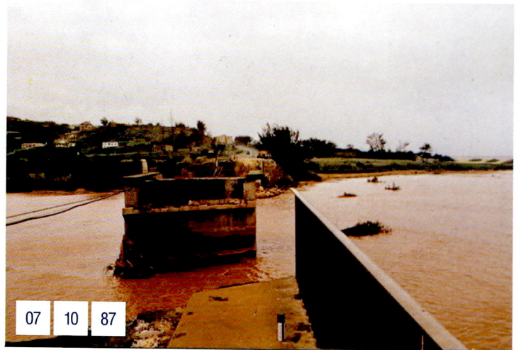
AFTER THE FLOOD
