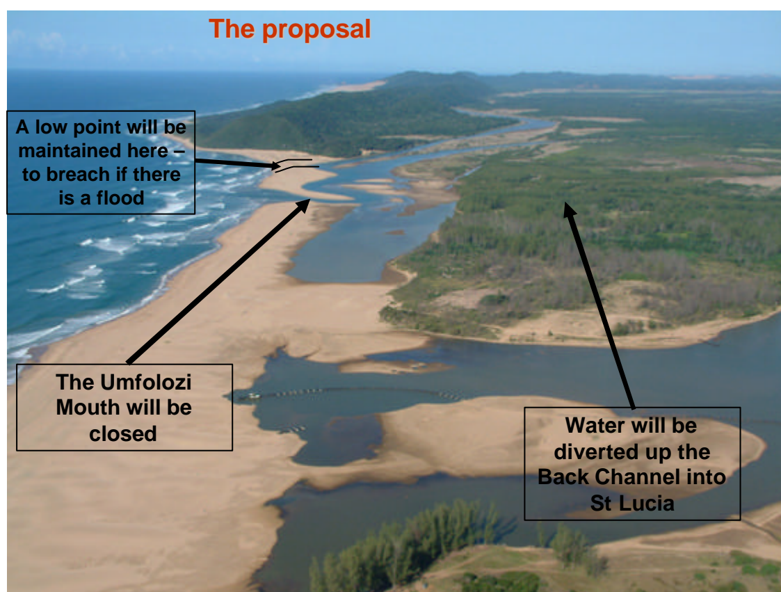
Figure 1. Layout of proposed plan to divert Umfolozi water into St Lucia (Photo provided by R.Taylor).
